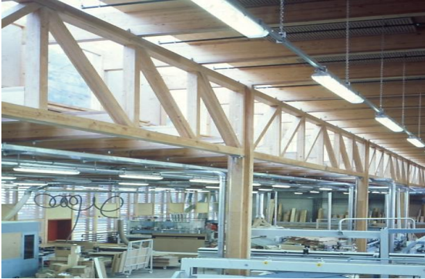
Figure 20: Truss girder: hardwood components connected with glued-in rods (2003)
